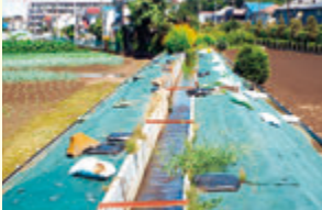
The canal helps you understand how the embankment was constructed to reduce the difference in levels of ground so that the water in the canals can flow.
