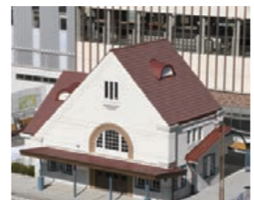
Restored triangular station building of the former Kunitachi Station
